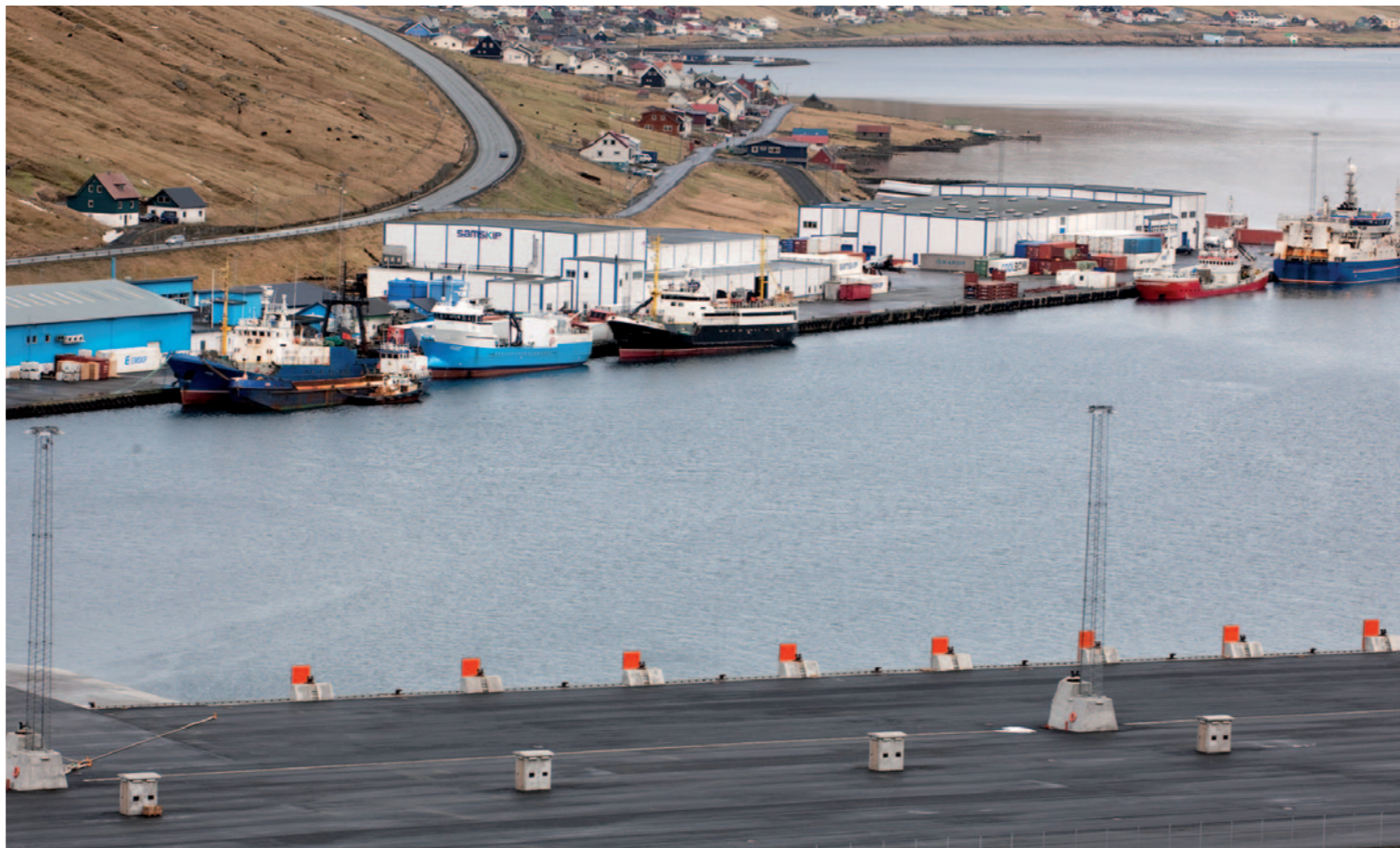
The Kollafjørður harbor with the new container terminal in the foreground; Tórshavn's East Harbour (bottom left); harbormaster Jónsvein Lamhauge (below).
