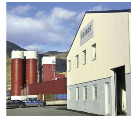
Bergfrost's head office with sorting hall.
