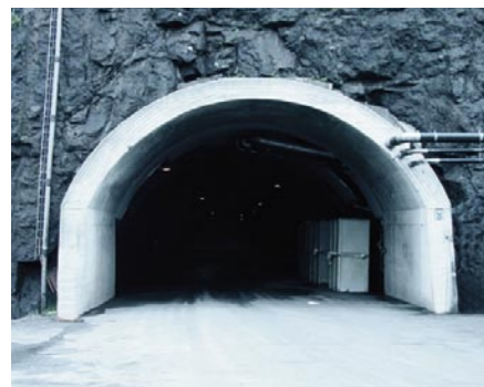
The entrance to the mountain tunnel (left); The mountain rock will make the storage temperature remain constant for a relatively long time in the event of operational disruption (right).
